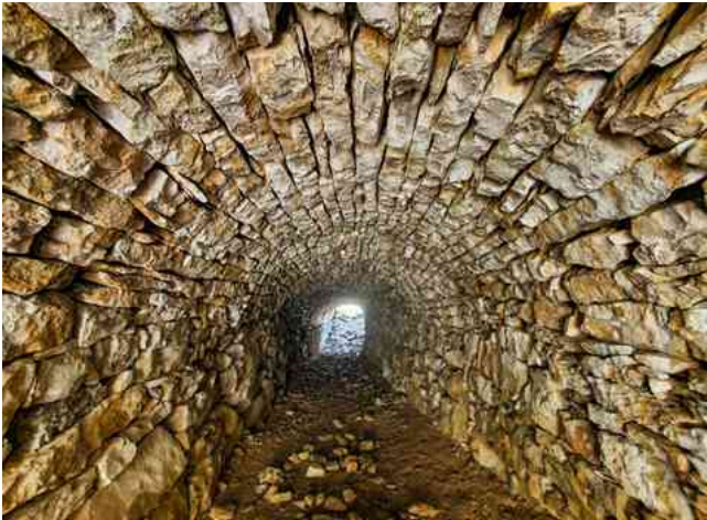
Tunnel de carrier (BL, 20/03/2024)
